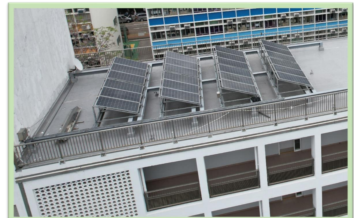
Installation of Solar Panels on the Rooftop of Kowloon Technical School
